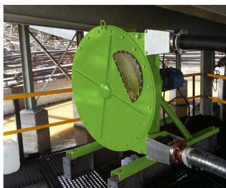
ALH100 for thickener underflow in mining industry
