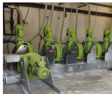
ALHX40 for lime slurry in wastewater treatment
