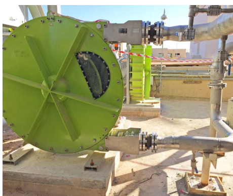
ALH125 pumping concrete
